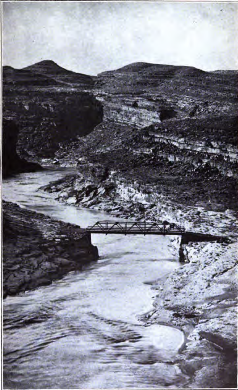
STATE HIGHWAY BRIDGE OVER SAN JUAN RIVER AT NARROWS, SAN JUAN COUNTY.
